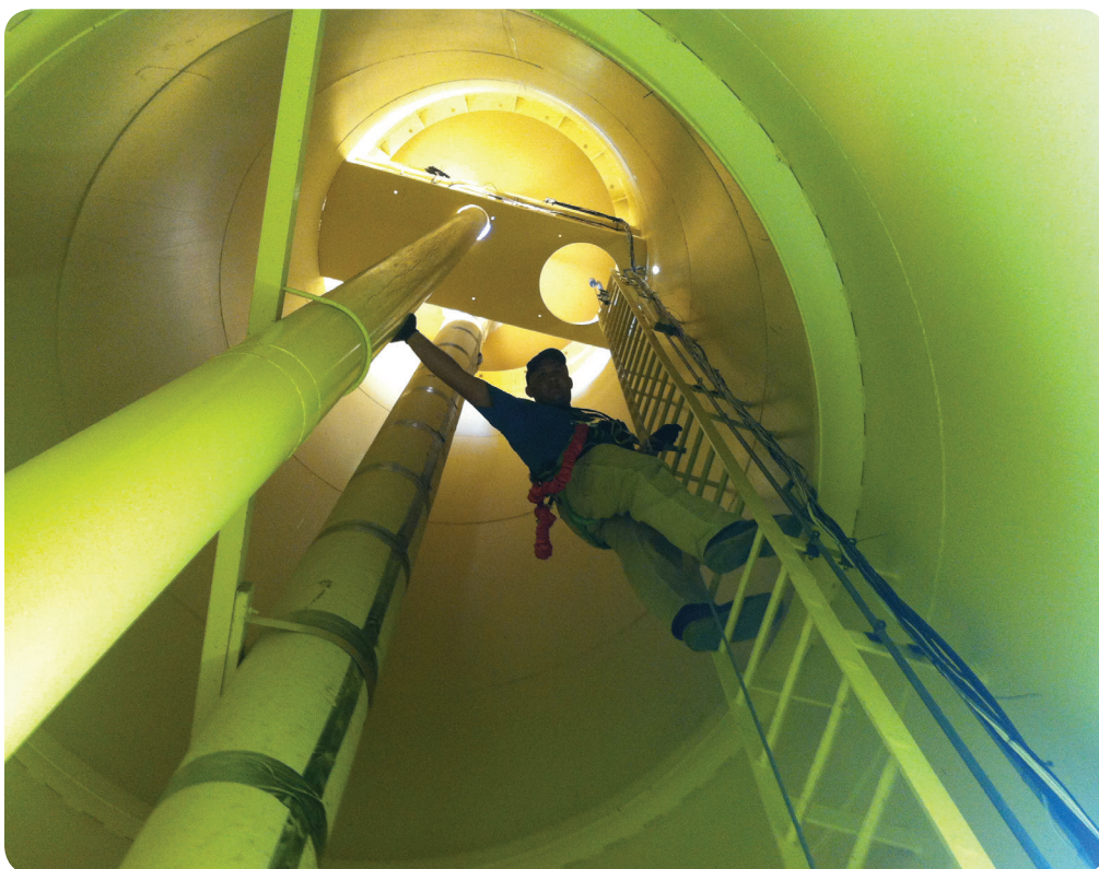
Above: Operations staff conduct inspections on Water tower piping
