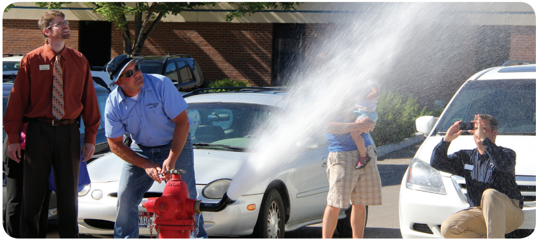
Above: Operations staff exercise and flush a fire hydrant
