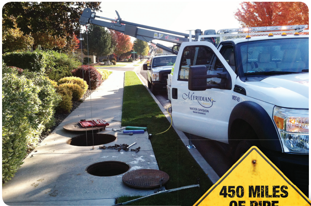
Above: Water production Staff conduct maintenance activities in an underground pressure regulating valve station.
